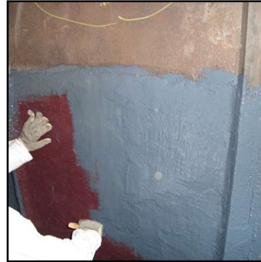
Belzona® 1391 provides a smooth surface and has the abrasion and temperature resistance required
