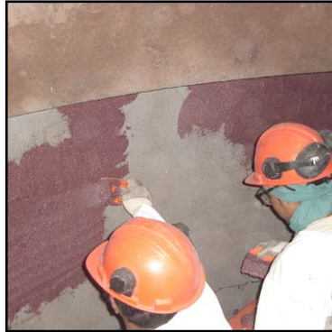
Belzona® 1811 (Ceramic Carbide) was applied to high wear areas to provide extra abrasion resistance
