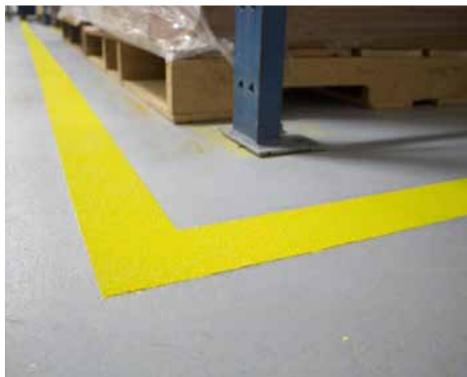
Used as a clear topcoat over Belzona 5231 and aggregate
