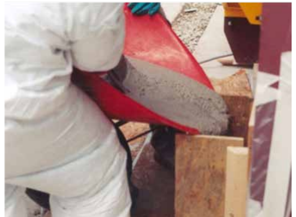
Belzona 7211 poured into place
