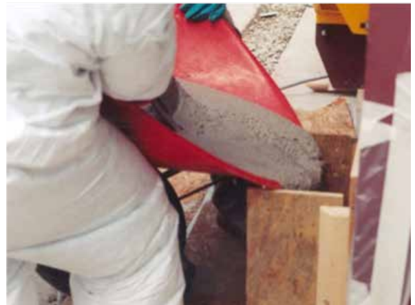
Belzona 7211 poured into place
