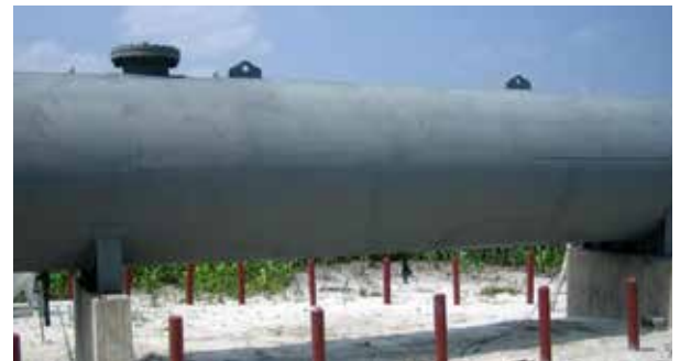
Vessel coated with Belzona 6111 providing a cathodic protection to the metal surface
