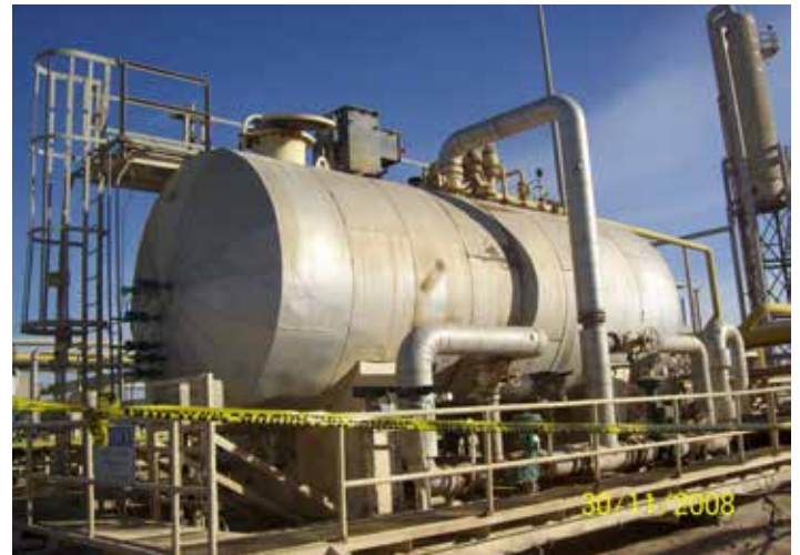
Belzona 5892 used to line a desalter
