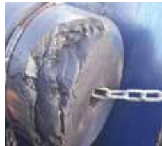
Damaged part rebuilt
