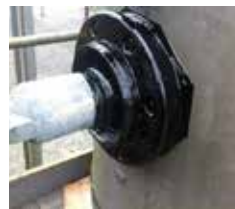
Transformers leak sealing
