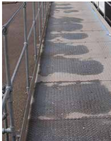
Polished steel ramp before coating
