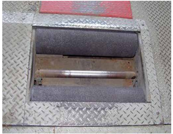
Drive Rollers - 12 years after the original application, still in excellent condition
