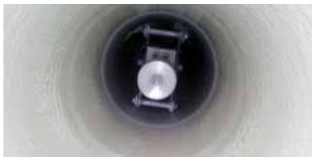
Before, during and after an application of Belzona 1381 being spin-sprayed on the internals of pipes
