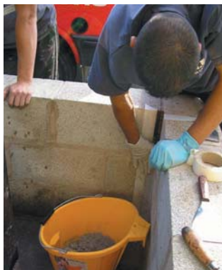
Fillets are added to give additional protection to corners
