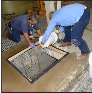
Reshaping the access opening
