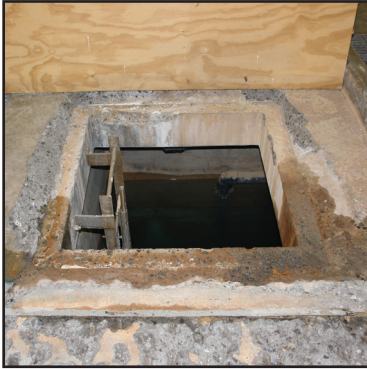
Floor prepared for resurfacing
