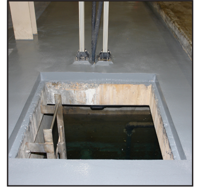
Rebuilt, protected, a first class job
