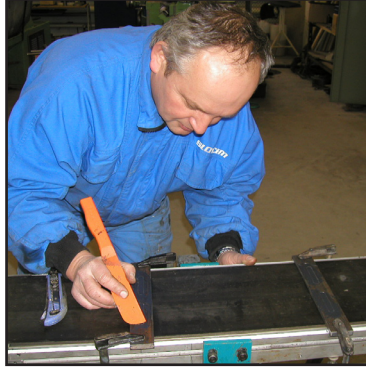
Application of Belzona® 2211
