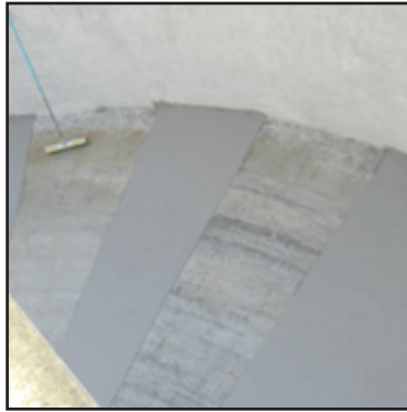
Application of Belzona® 4111
