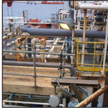
Belzona® 5851 applied to exposed pipe work
