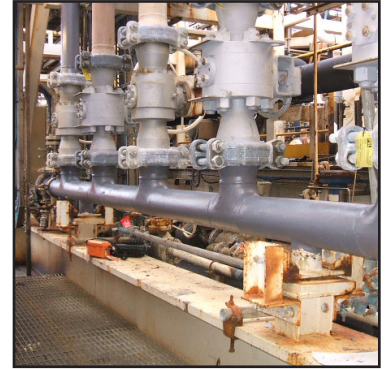
Belzona® 5851 applied to the Manifold
