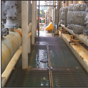
Belzona® 5851 applied to exposed pipe work
