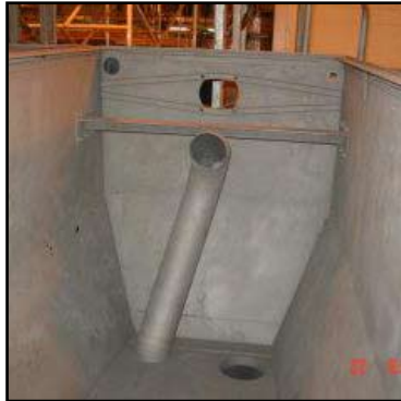
Blasted ready for repair and coating
