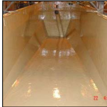
Belzona® 5811 first coat complete
