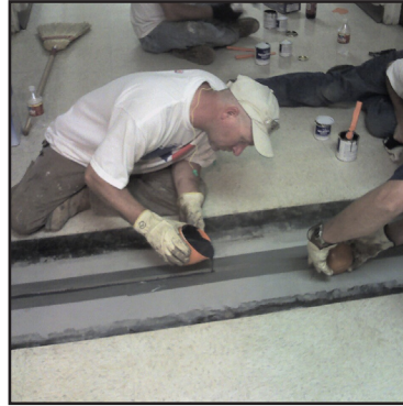
Application of Belzona® 2221
