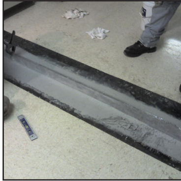
Application of Belzona® 4111
