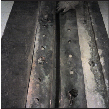
View of joint with kick plate removed
