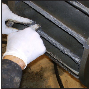
Rebuilding and reinforcing with Belzona® 1111
