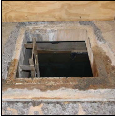
Floor prepared for resurfacing
