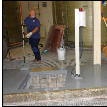
Belzona® 5811 Grey coat over Beige with Surefoot added
