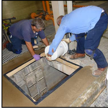
Reshaping the access opening
