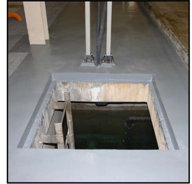
Rebuilt, protected, a 1st class job
