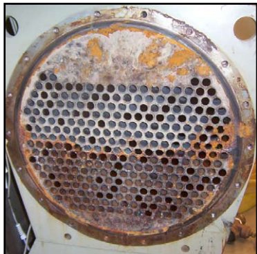
Tube sheet before blast cleaning.
