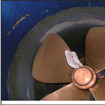
Localized damage to Belzona® 1341 (Port)
