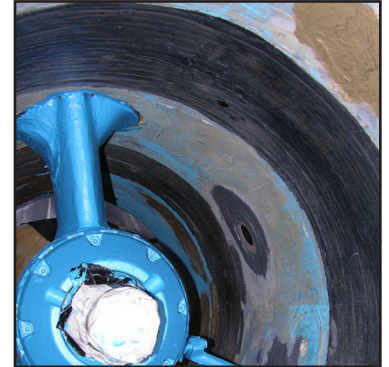
Inspection after 5 years service
