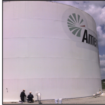
View of tank size
