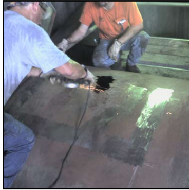
Surface preparation underway
