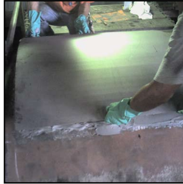
Doubler plate being positioned and bonded in place
