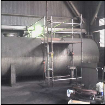
General view of the tank
