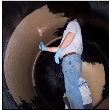
Contractor applying 2nd coat of Belzona® 5811
