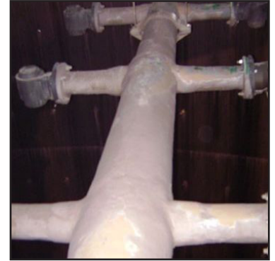
Belzona repair after seventeen months in service
