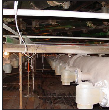
Completed Belzona application to one of six lime slurry header pipes
