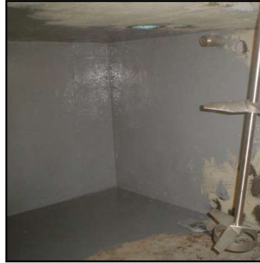
First coat of Belzona® 5811 being applied
