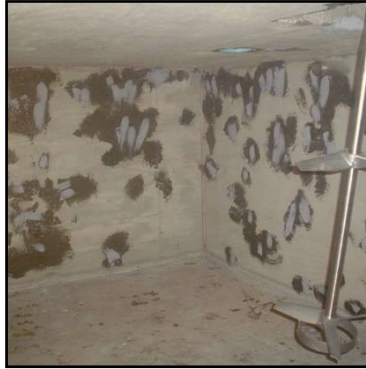
Surface prepared and holes patched with Belzona® 4111
