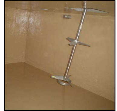
Final coat Belzona® 5811 applied
