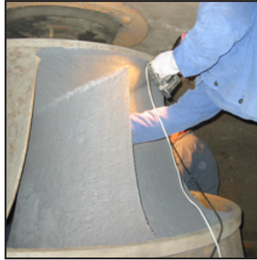
Rebuilding with Belzona® 1111
