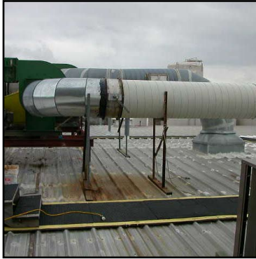
First duct joint
