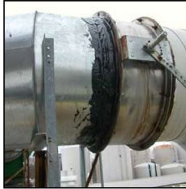
Close up of first joint repair
