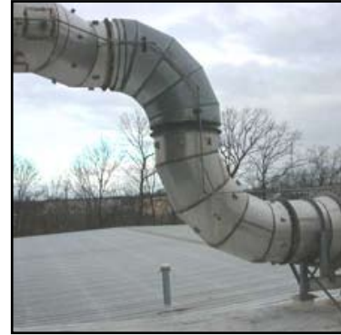
Second joint repair
