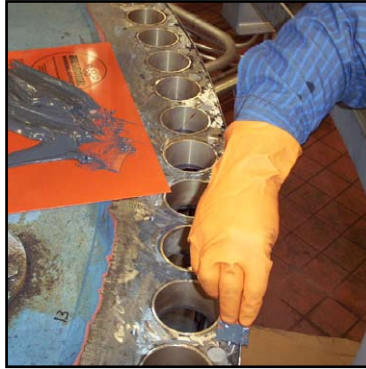
Surface restoration with Belzona® 4301
