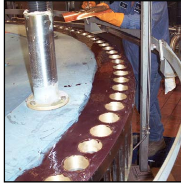
Surface coated with Belzona® 4311
