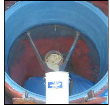
Second coat of Belzona® 1341 applied to complete the application.
