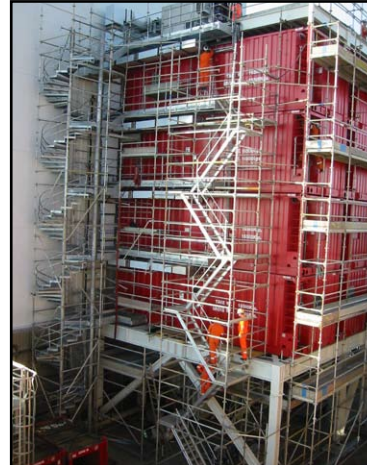
Accommodation Modules in position.
