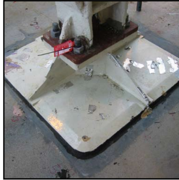
Bonding application completed.
