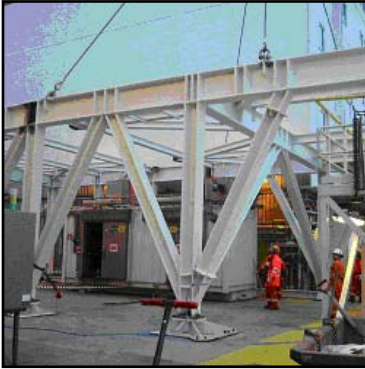
Lowering of sub frame into position and alignment.
