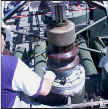
Surface preparation in progress
