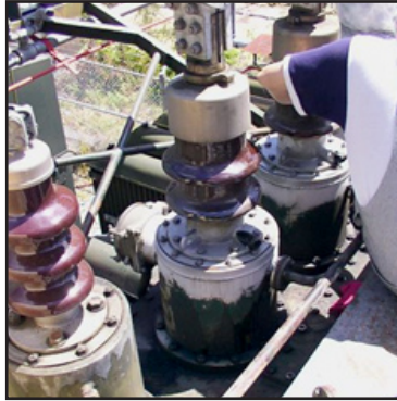
Surface preparation by grit blasting completed
