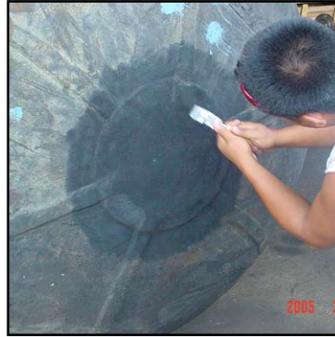
Surface preparation for the fender.
