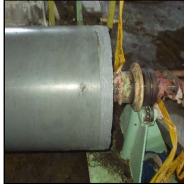
Belzona® 1111 applied to the roll
