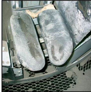
Condition of the coated steel plate and steel seat after one year in service.
