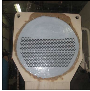
Tube sheet completed.
