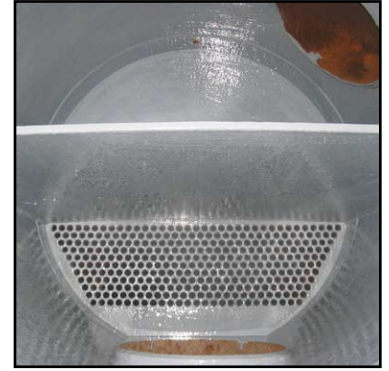
Water box completed.
