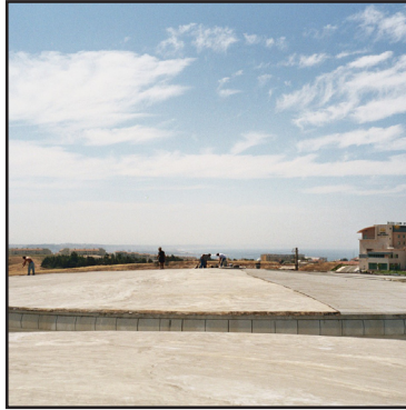
Preparation of roof surface
