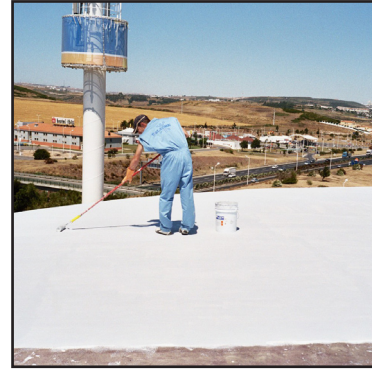
Application of Belzona
