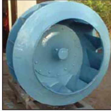
Second coat of Belzona® 1341 completed on fan
