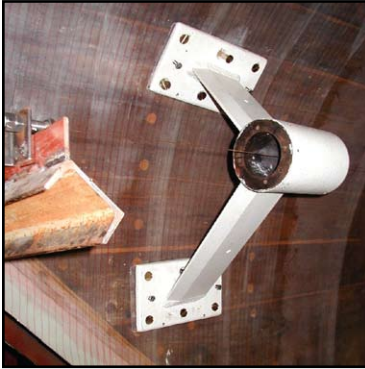
Bracket positioned using aligning wire and jacking bolts.
