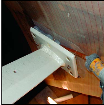
Belzona ® 1121 being injected between hull and bracket.
