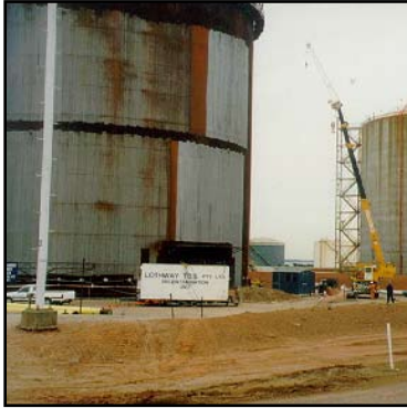
General view of the tank
