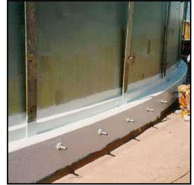
Application being completed
