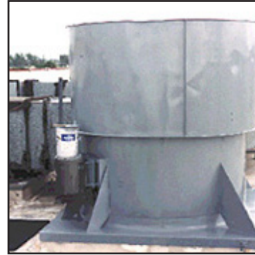
Completed coating with Belzona® 5111 (Ceramic Cladding)
