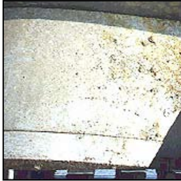
Cavitation damage to stabilizer trailing edge.
