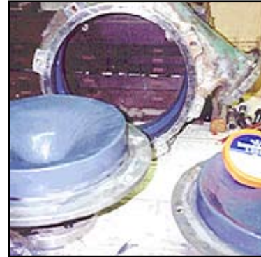
Rebuilt and coated lime sludge pump
