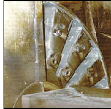
Two coats of Belzona® 1321 for a finished smooth surface
