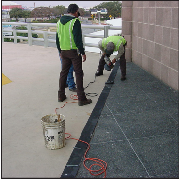
Joint before - showing old system
