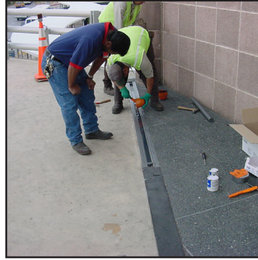
Belzona® 2221 being poured into joint
