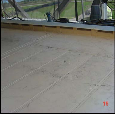
Roof over cascade area prior to the application (note seams).
