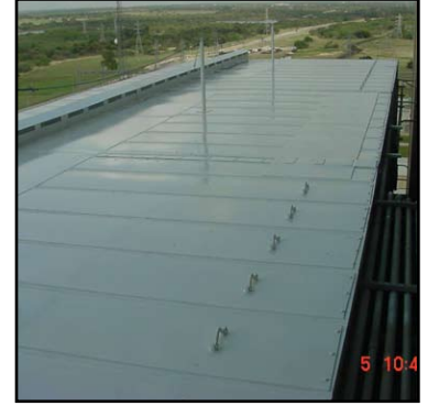
Completed roof. (Roof was painted following the application of the Belzona.)
