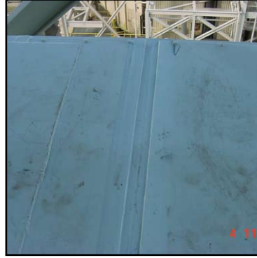
First coat of Belzona® applied.
