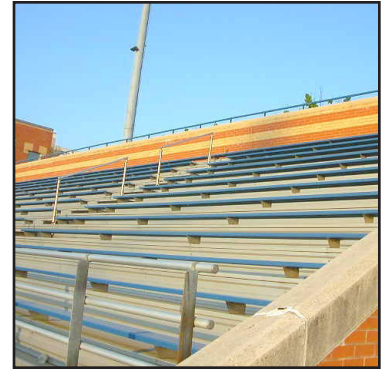
Completed north wall area
