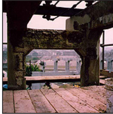
Work carried out from simple scaffold platform
