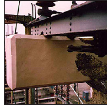
Close-up of a rebuilt beam prior to application of Belzona® 5151
