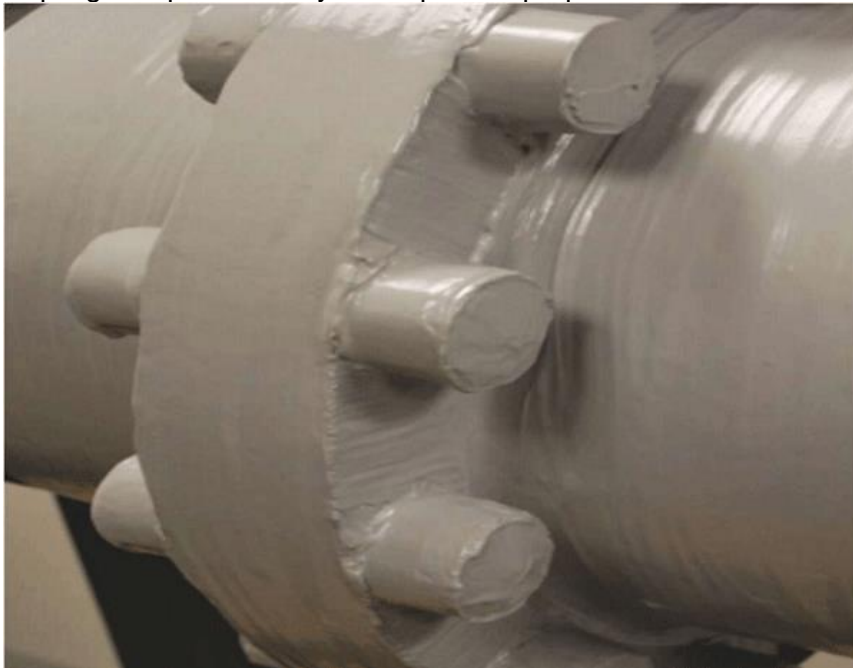
Figure 1: An encapsulating system protects a flange.
