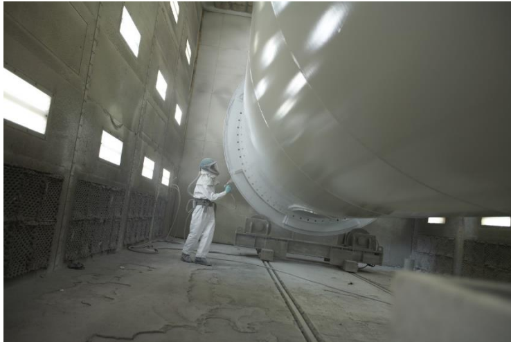
Hazardous spraying applications require correct protection, including respirator
