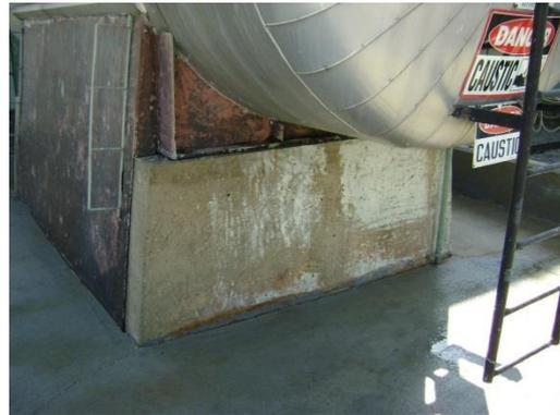
Fig 1 and 2 – Examples of deteriorated secondary containment
